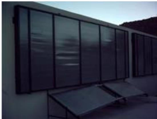
FIGURA 23: Colectores de Aire, Hospital Susques Jujuy
