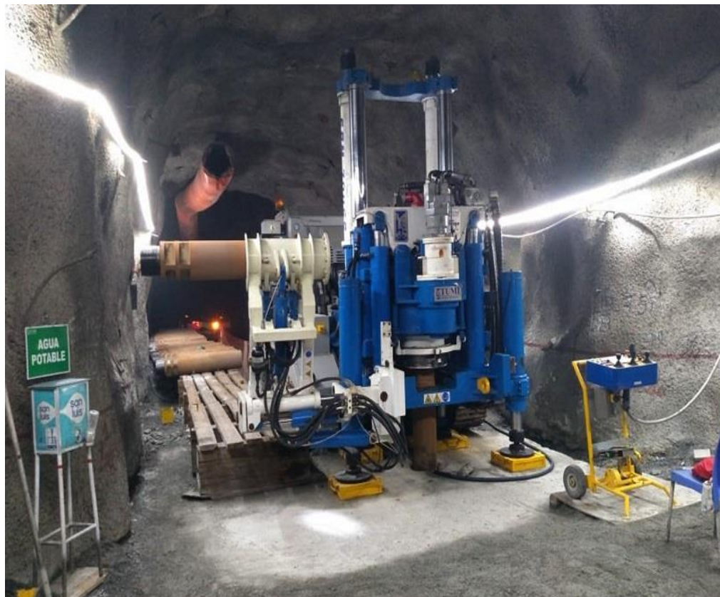
Figura 1. Raise Boring: La SBM 700 SR
