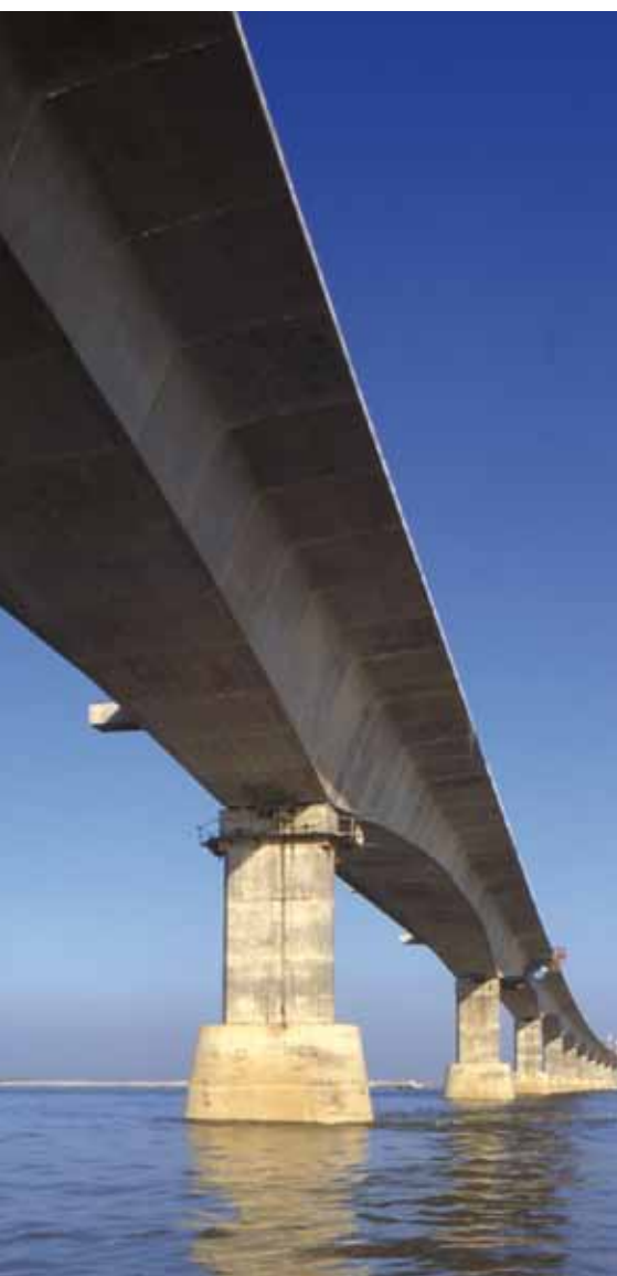
Jamuna Bridge, Bangladesh
