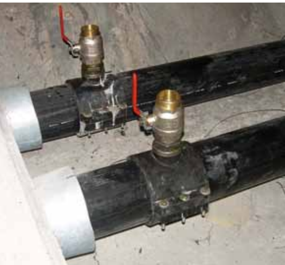
Injection inlets on HDPE pipes
