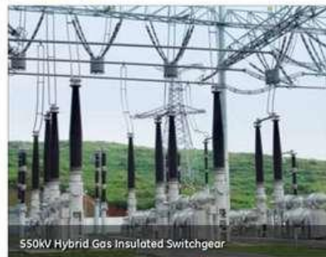
550kV Gas Insulated Switchgear
