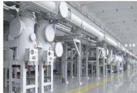
550kV Gas Insulated Switchgear
