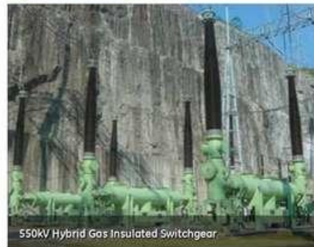
550kV Hybrid Gas Insulated Switchgear
