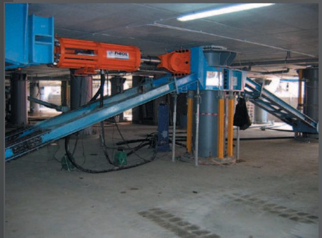
• Dynamic tests on a building of the C.A.S.E. project in L'Aquila (Italy) isolated with FIP-D devices.
