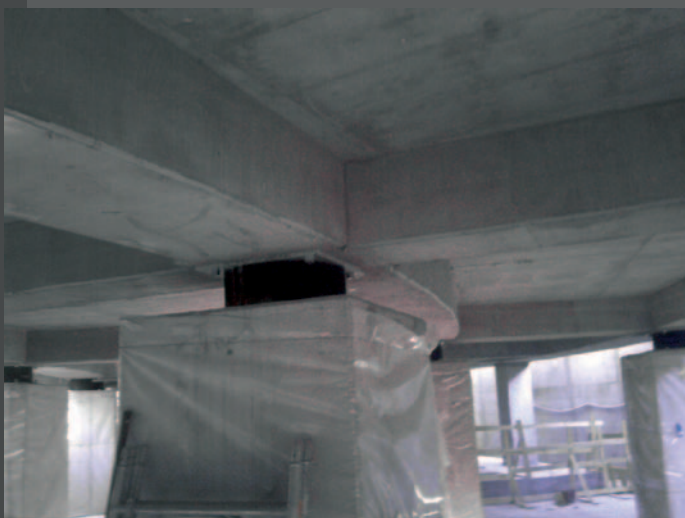
• L'AQUILA, ITALY - ANAS new Head Office: installation
