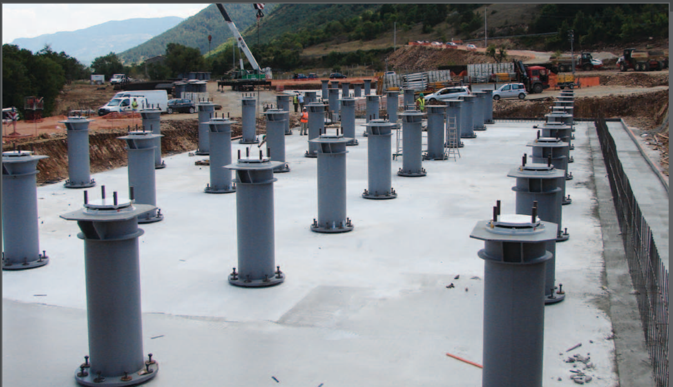
• L'AQUILA, ITALY - C.A.S.E. Project, installation of FIP-D
