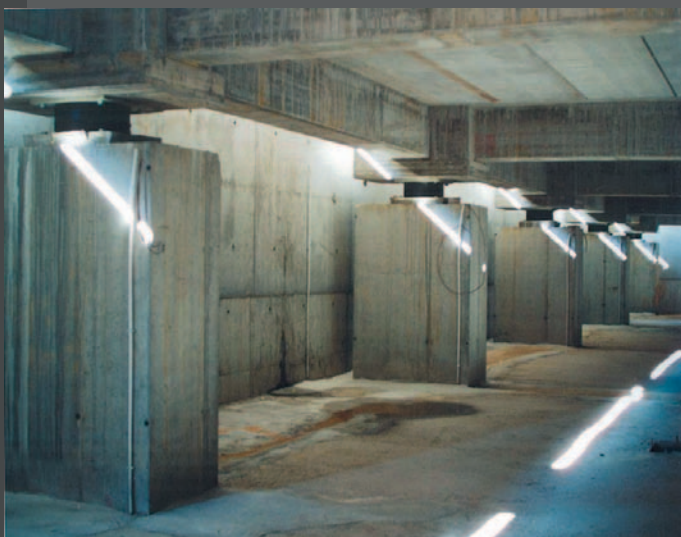
UDINE, ITALY - "Gervasutta" Hospital: installation
