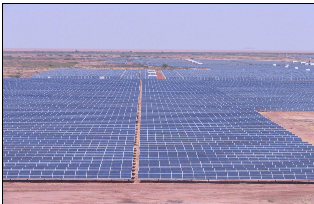
Figura 17: Charanka Solar Park. 345 MW. India.
